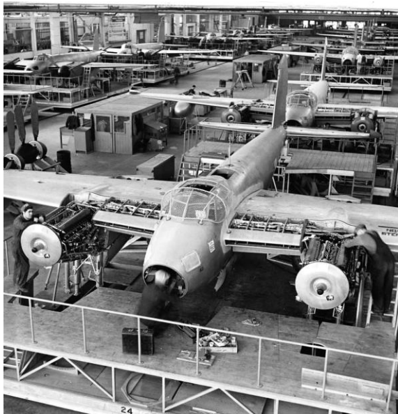
A Mosquito being assembled at the Downsview Plant. Source: www.facebook.com/groups/112232095483062/posts/27166087186337520/
