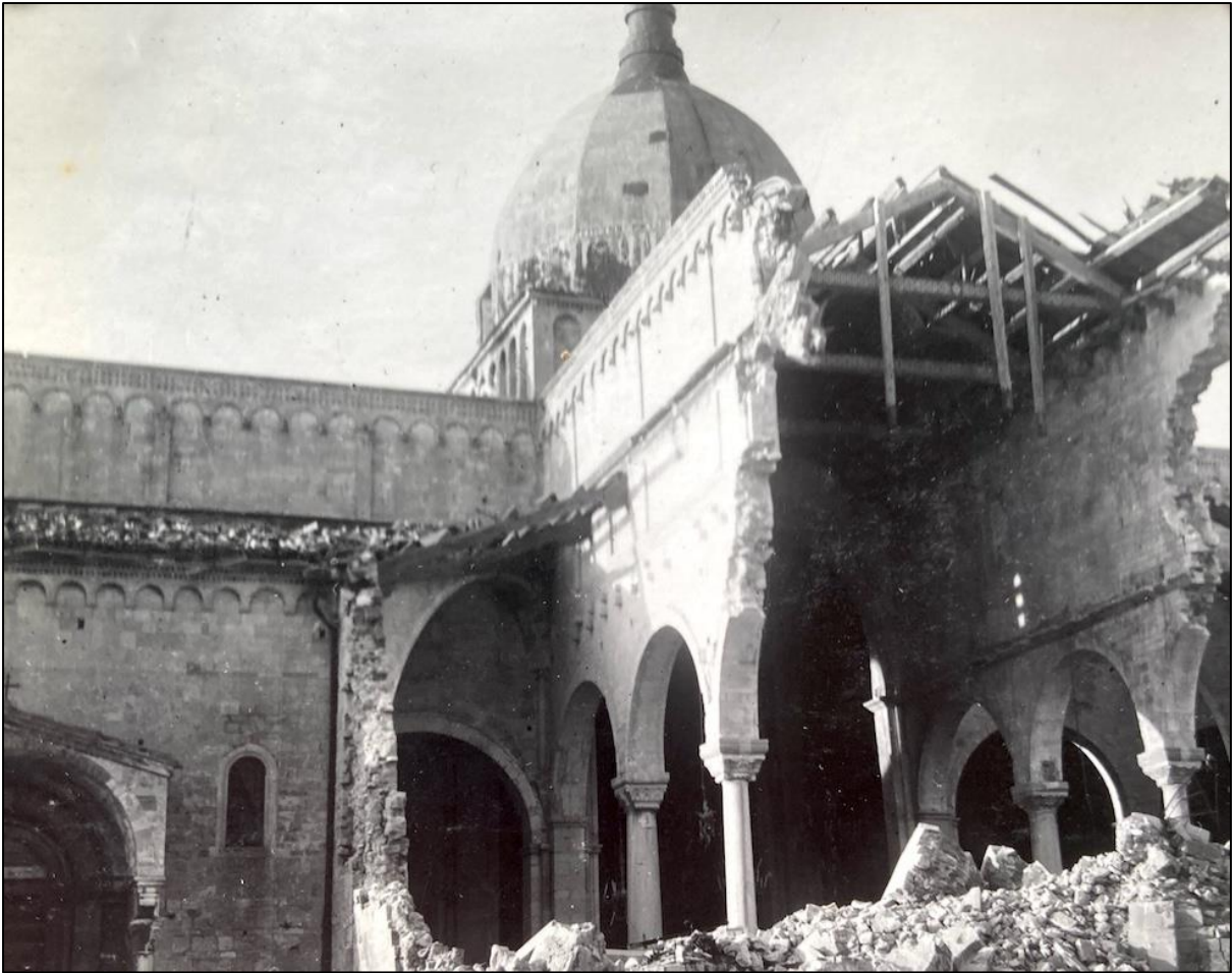
Damaged Ancona Cathedral.
